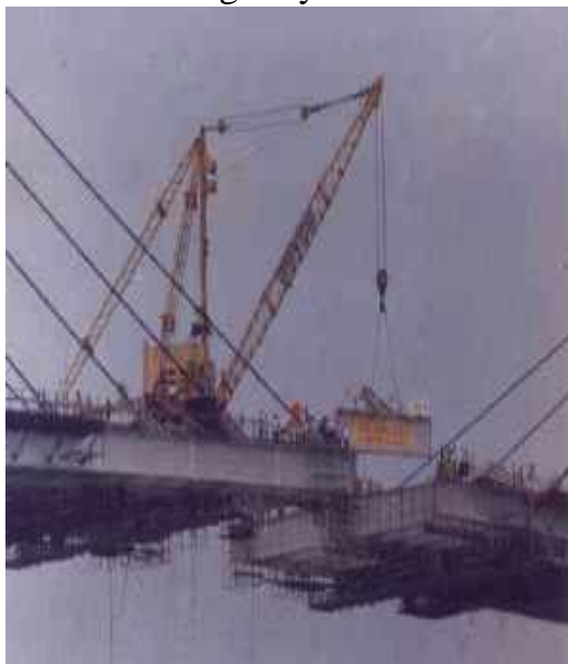
Figure 4. The mid-portion of the deck of the Second Hooghly Bridge being constructed, vividly showing some of the high capacity cranes used
