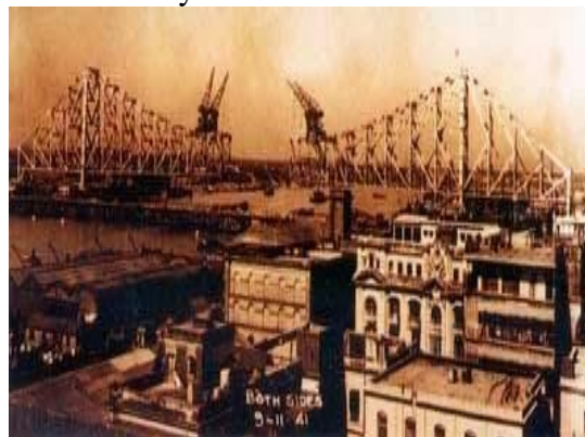
Figure 3. Howrah Bridge under construction
