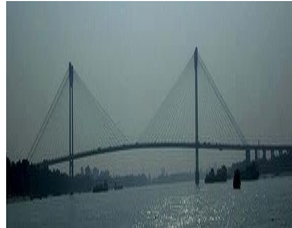
Figure 2. View of Second Hooghly Bridge, as seen from Howrah Bridge.
